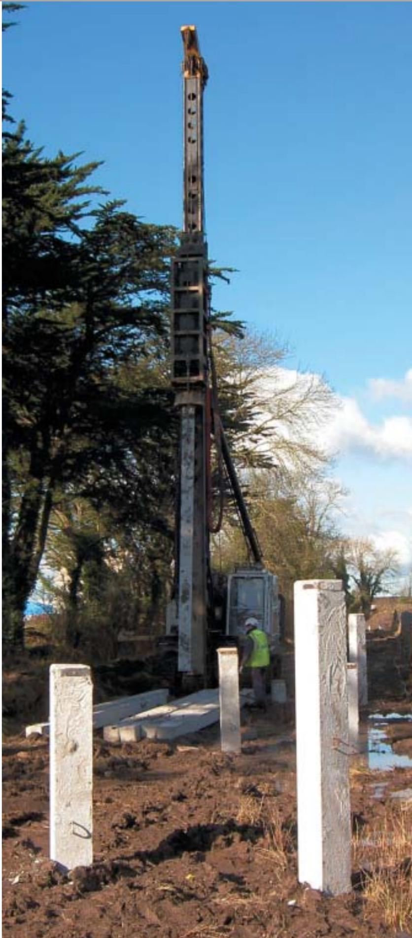
**Driven Piles provide a choice of materials - they can be; Concrete, Steel, Timber, Composite**
